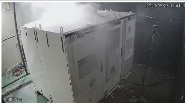
Figure 14: During thermal runaway (Time at 17:41)
