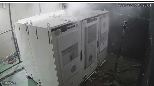
Figure 19: 3 rd thermal runaway (Time at 18:25)
