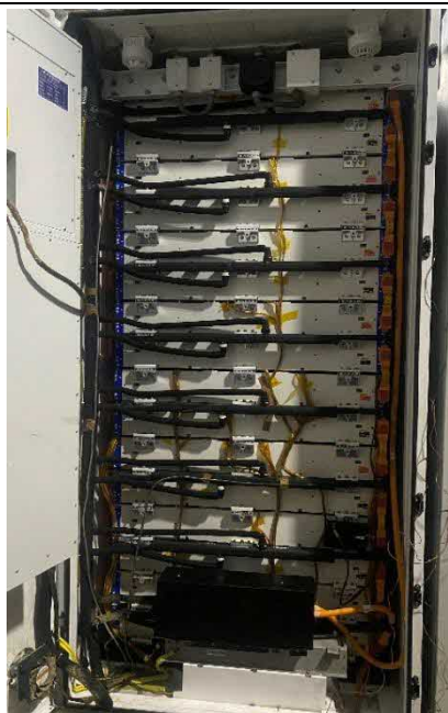
Figure 3: BESS unit internal view(Front)
