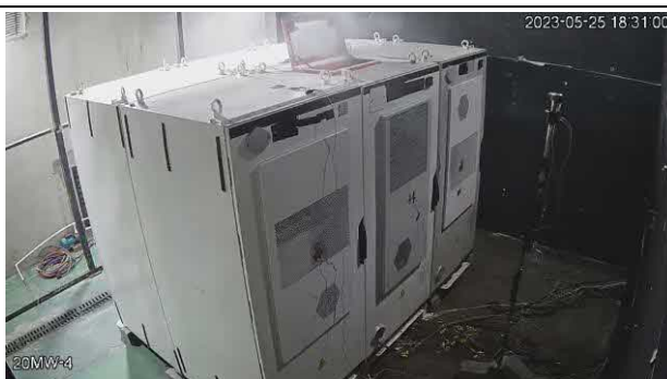
Figure 20: 4 th cell venting (Time at 18:31)
