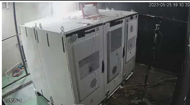
Figure 22: 4 th thermal runaway (Time at 19:10)
