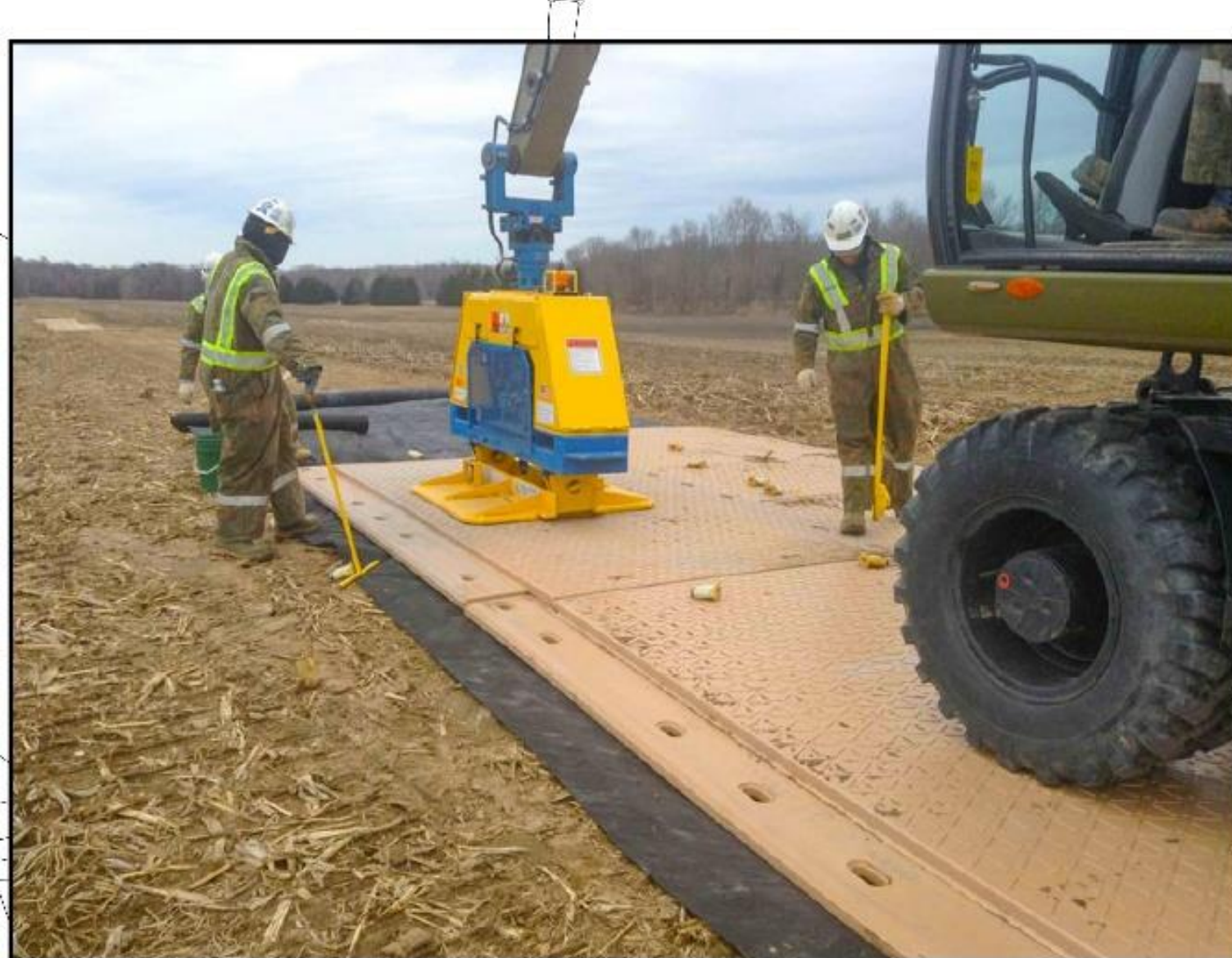
The haul route will be built by laying ground protection mats on the top of the grass in the fields. The access onto the East Claydon Road will be gated and will comply with highway regulations. On completion of construction the boards will be removed, the farmland restored and hedge gaps replanted.
